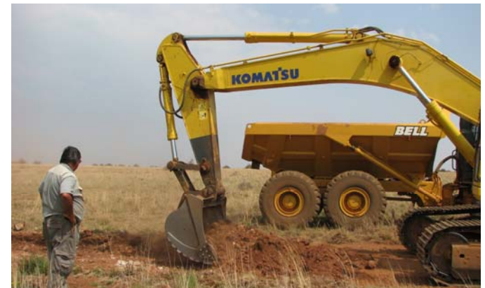
Mining of surface gravel
